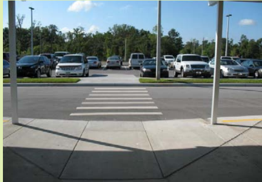
Not all sidewalks have curb ramps on both sides of the crosswalk
